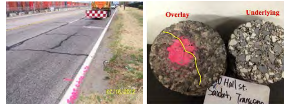
Figure 2. Pavement Condition of WMA Pavement (left); Field Core at Tip of Transverse Crack (right)
