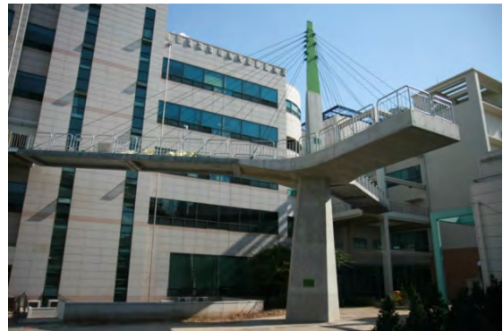
UHPC pedestrian cable stayed bridge built at KICT
