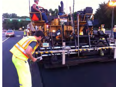
Figure 2. LEADCAP pavement during night construction of State Highway TH 169 in Minnesota
