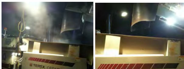
Figure 1. HMA (left) and LEADCAP (right) mixes during night construction of State Highway 6 in Iowa
