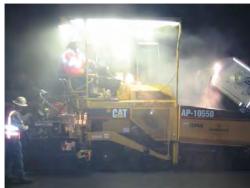
Figure 1: Smoke from HMA during night paving
