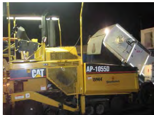
Figure 2: Smoke elimination with WMA during night paving
