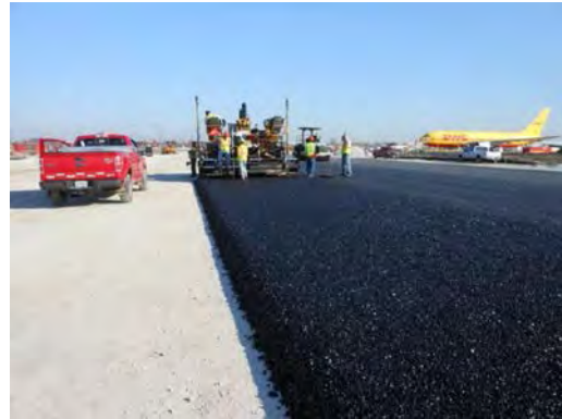
Figure 2. Rediset LQ warm mix paving of Taxiways at O'Hare Airport in Chicago
