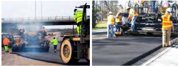
Figure 1. Standard HMA (left) and Rediset WMX (right) paving of US 190 between Jasper and Woodville, TX.
