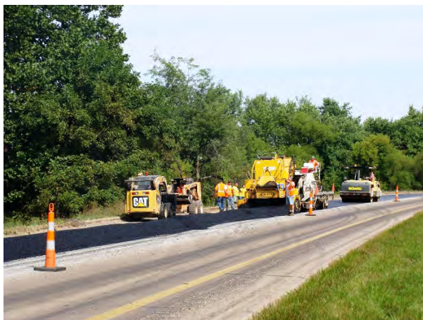
Henningsen Construction paving WMA
