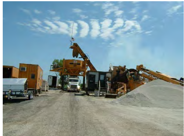
Asphalt Plant running Warm Mix Asphalt
